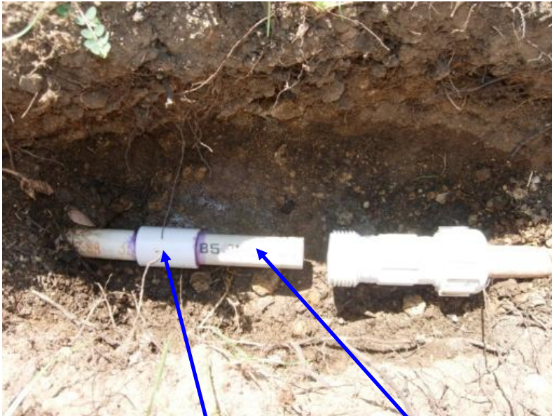
Solvent weld socket coupling and pipe stub
