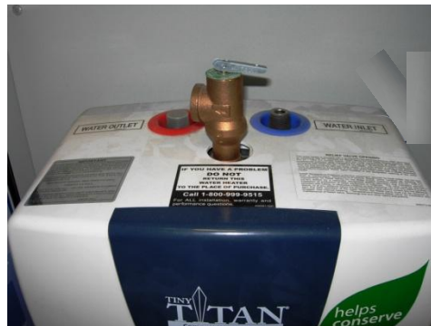
Tankless Heater TPR Valve
