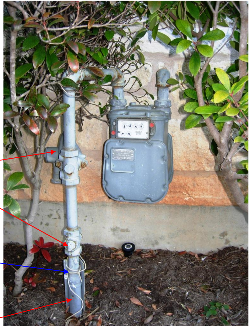
Typical Natural Gas Connection
