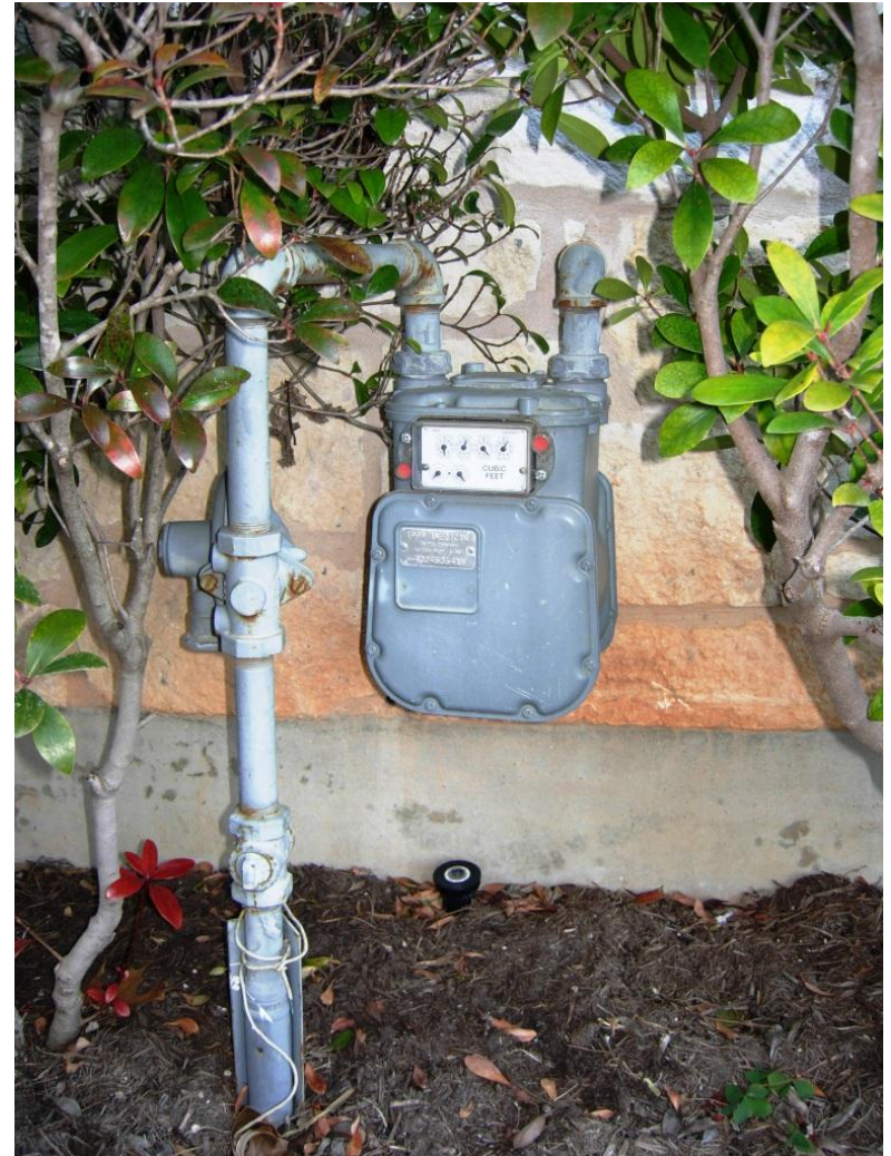
Typical Natural Gas Connection
