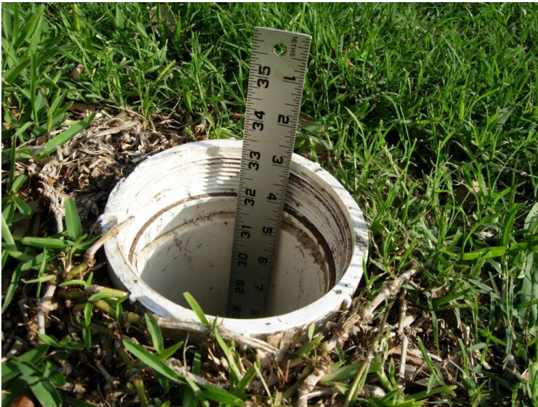
Typical Sewer Cleanout
