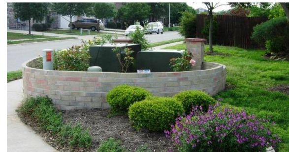
Examples of Utility Box Screening
