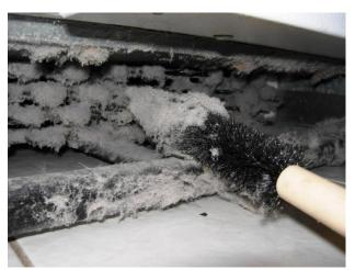
Use the vacuum hose to remove debris from the brush with each pass through the coils.
