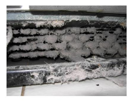
The basic idea is to get all the dust and dirt out from among the coils without damaging them. The coils are fairly robust but could be damaged by sharp or stiff tools.
